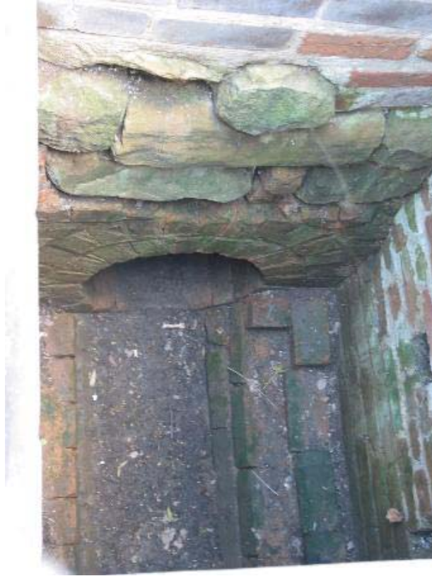
The drainage pit at the back of the Ranger's Cottage, which carried the slops washed from the dairy. The slightly lower level of the drain before entering the pipe probably allowed sediment to settle for later extraction before liquids entered the river.
