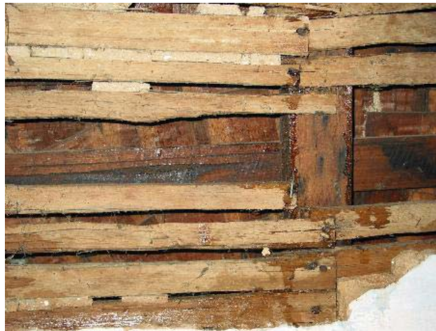
Lathe and plaster ceiling, under the wooden shingled roof, show remnants of plaster “keys” pushed through the timber to hold the plaster in place.
