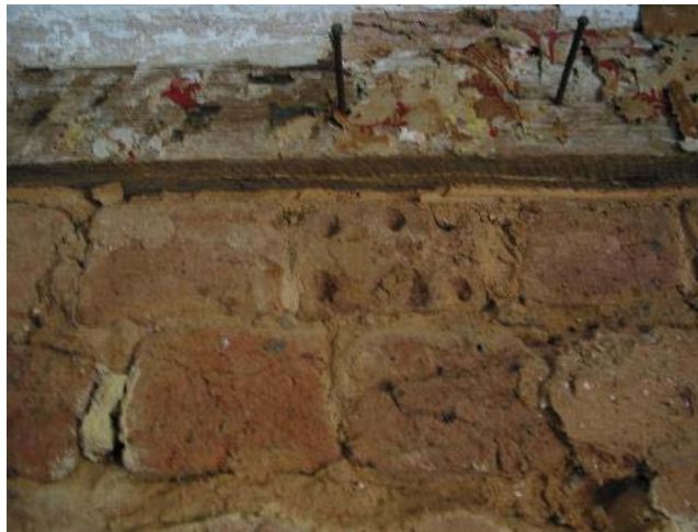
In rooms added to the original cottage, handmade bricks reveal tally marks, where fingers were stuck into the clay to mark completion of a set number – probably 100.
