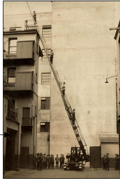
Figure 11 – View of rear yard facing south, showing the stables following conversion into an engine bay. The second storey has been removed and a flat roof erected over both the stables and passageways. Note the vehicular entrance in the rear wall of the stables, (circa 1920s), NSW Fire Brigades Historical Archive (uncatalogued).
