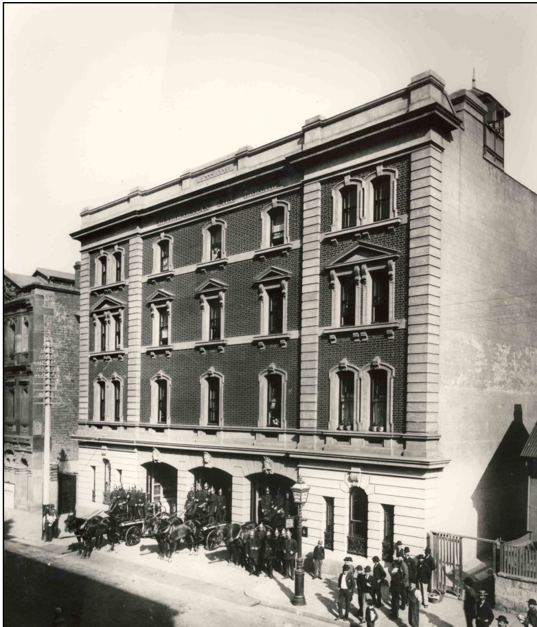
Figure 2 – The opening of Central Fire Station (1888). Note the watchtower on the roof, which was set back from the façade to facilitate symmetry following revision of the plans by Barnet at the Board's request. Note also the cottage to the right, NSW Fire Brigades Historical Archive (uncatalogued).
