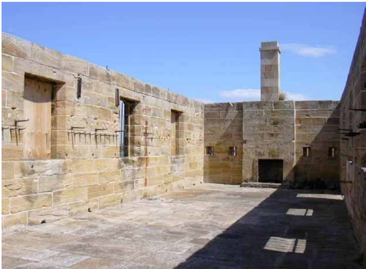
Empty, roofless and silent, the convict guardhouse at Cockatoo Island nevertheless speaks volumes. Built by convicts under duress, the stone walls bear witness to the sadistic cruelty of one of the overseers who made his charges remove 160 pegs they had fitted into the walls and replace the same pegs lower down. Photo R Broomham
